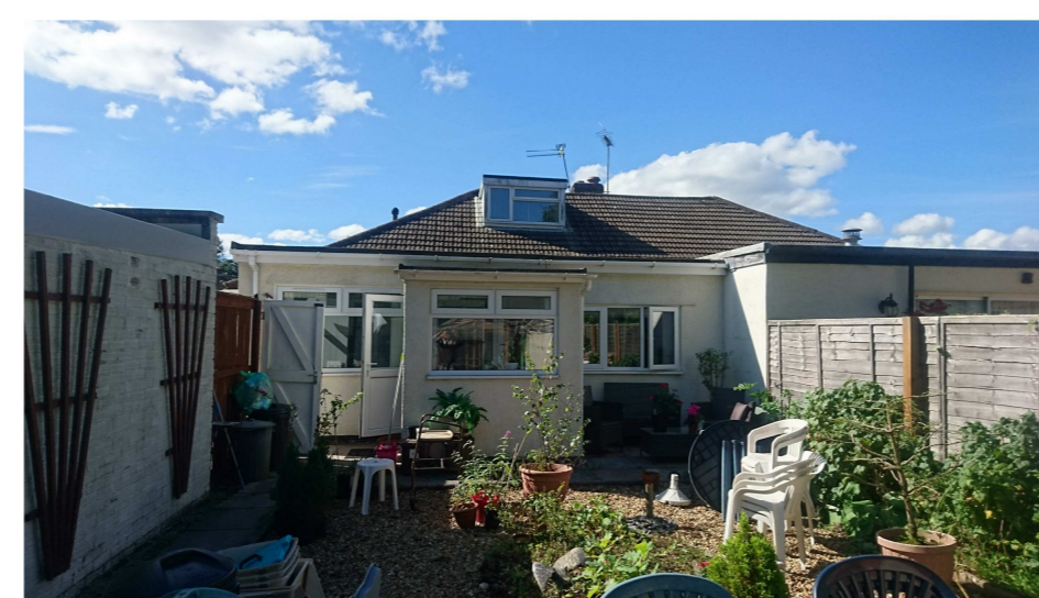
Existing Rear Elevation Image 1
