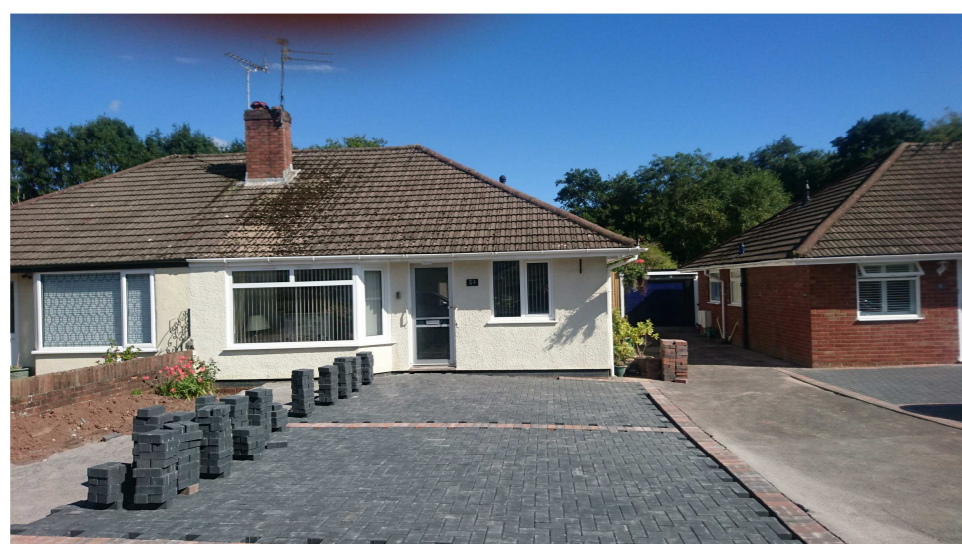
Existing Front Elevation Image 1
